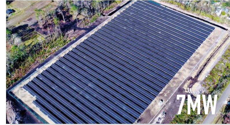
Project Type: G-Mounted Location: USA / Florida Commission Date: 2017-12 Product: SRP-325-6PA
