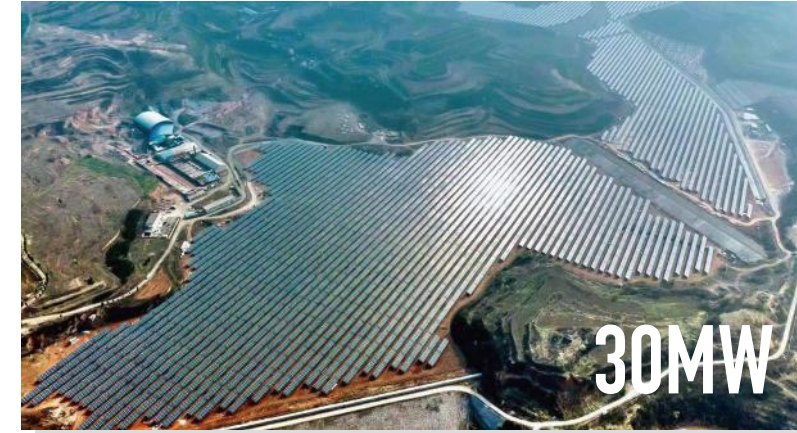
Project Type: G-Mounted Location: China / Shanxi Commission Date: 2020-12 Product: SRP-440-BMB-HV
