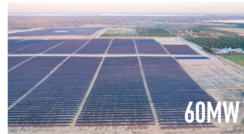
Project Type: G-Mounted Location: USA / Florida Commission Date: 2020-1 Product: SRP-365-6MA
