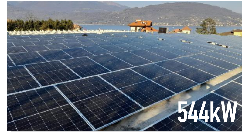
Project Type: Commercial Rooftop Location: Italy / Baveno Commission Date: 2023-10 Product: SRP-415-BMD-HV
