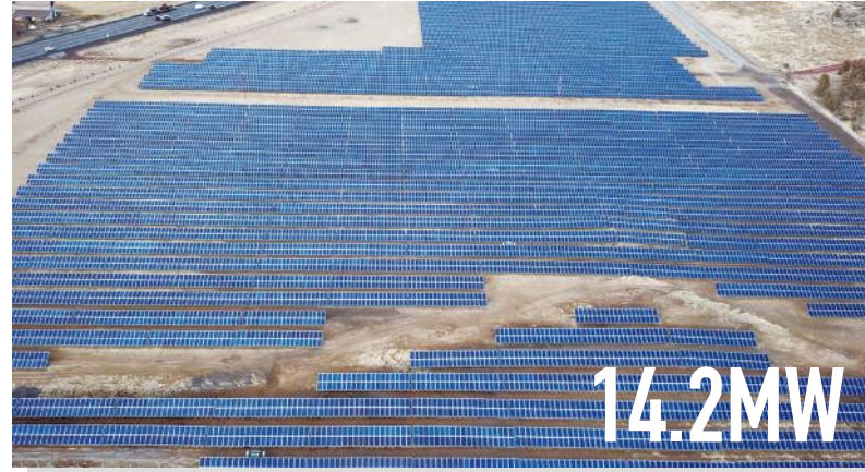
Project Type: G-Mounted Location: USA / Oregon Commission Date: 2017-11 Product: SRP-325-6PA
