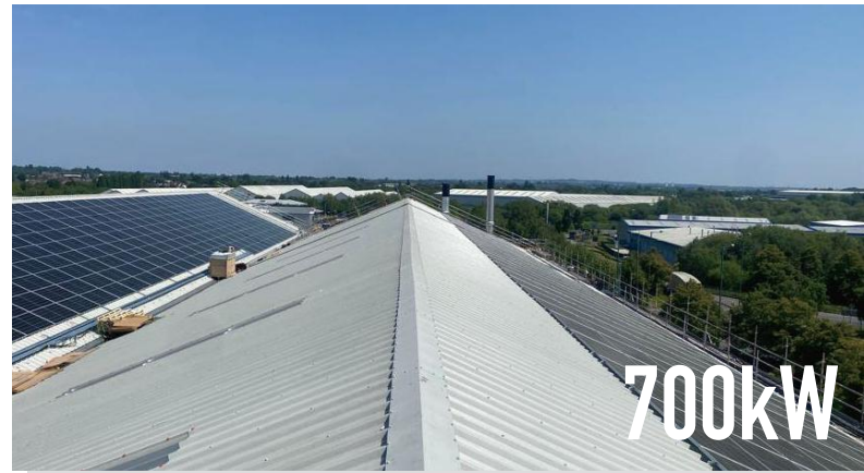
Project Type: Commercial Rooftop Location: UK Commission Date: 2023-6 Product: SRP-550-BMA-HV
